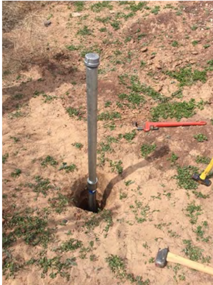
Figure 2-1. Attempt at Well Point Installation - Proposed Discharge Point
