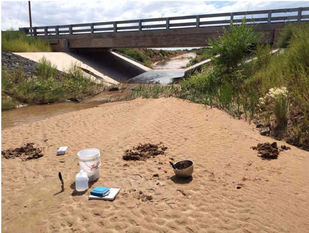
Figure 2-9. Location RSJ #7 Looking Downstream towards Nimitz Rd. Bridge
