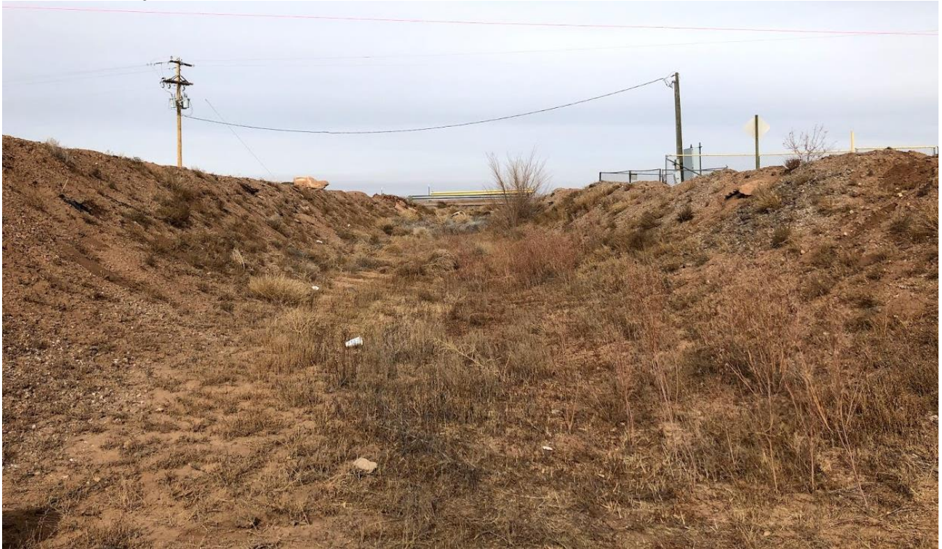
Looking Upstream at location of Cross-Section, Parallel to Flow
