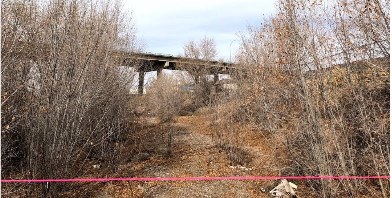
Looking Upstream at location of Cross-Section, Parallel to Flow
