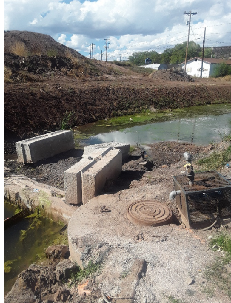
14. Dam downstream from RSJ#5, October 8, 2019 Photo from INTERA, Bryce Williamson
