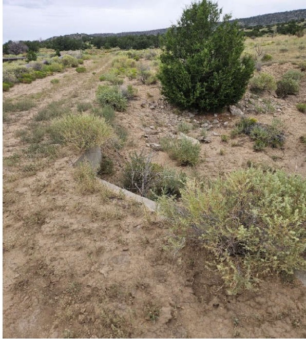
Photograph 1 – Concrete Wing Walls for an Arroyo Crossing
