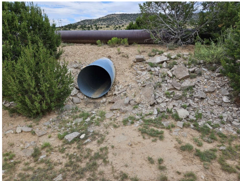
Photograph 2 -CMP Arroyo Crossing Under the Discharge Pipelin
