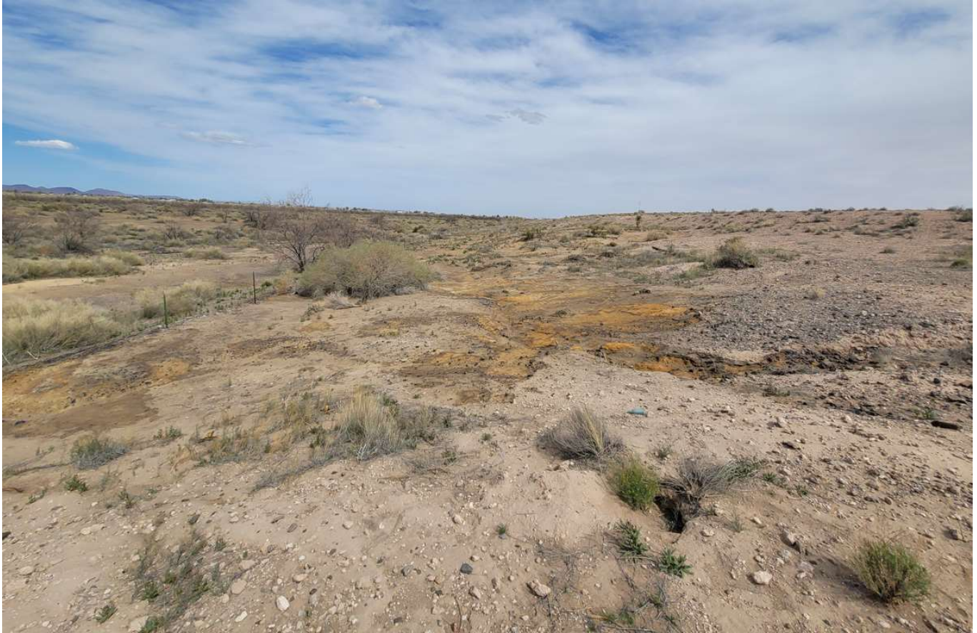
Figure 13. Cypress North Slope Reclamation Cover material erosion and tailings dispersion.
