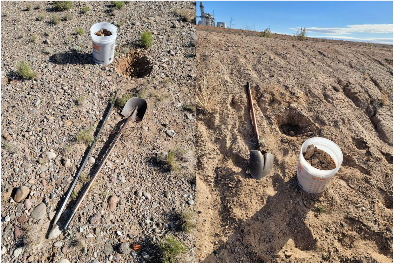
Figure 17. In-bank Gravel Cover and Fine Cover Material in borrow pit.
