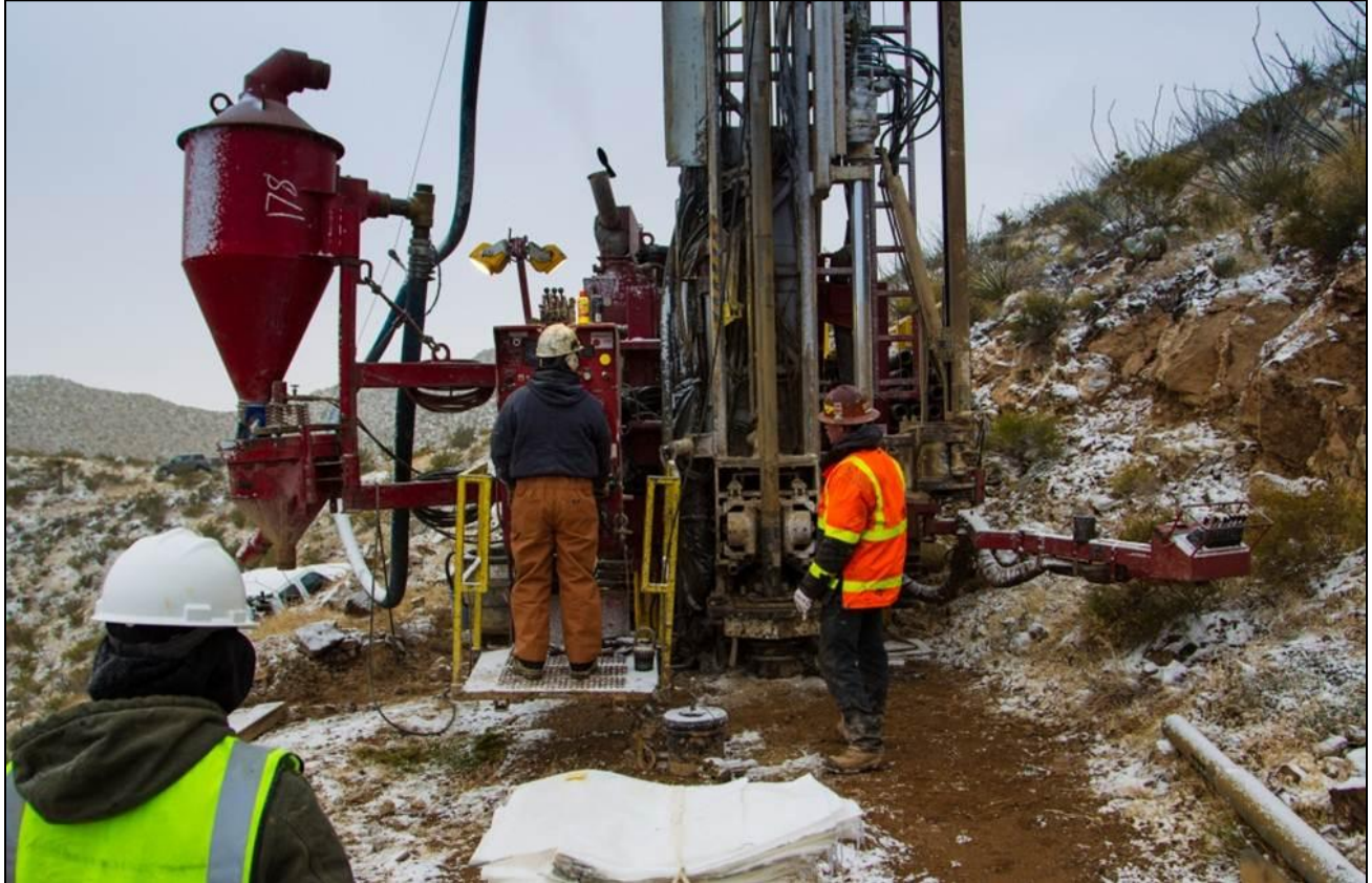
Figure 3: View of drilling of hole Tt-05
