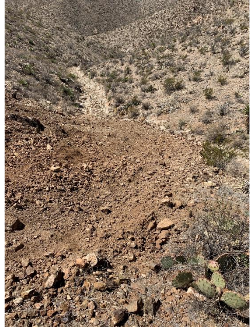
FIGURE 4 FROM MID-POINT DOWN THE SLOPE, LOOKING INTO THE ARROYO
