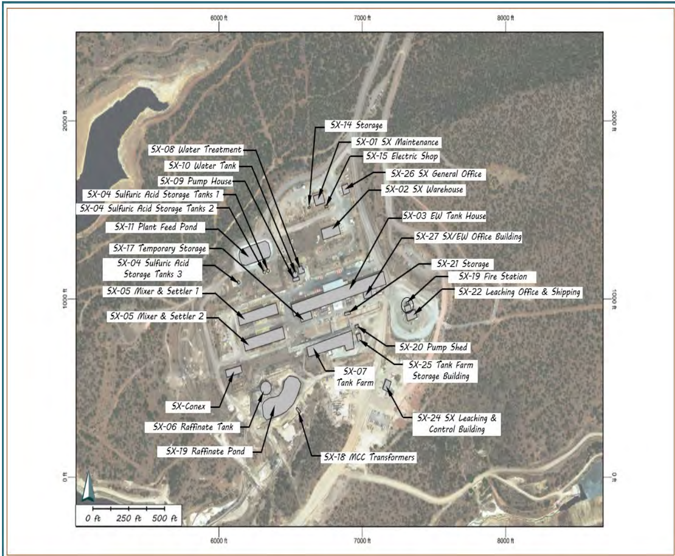
Figure 2 SX/EW Area Buildings
