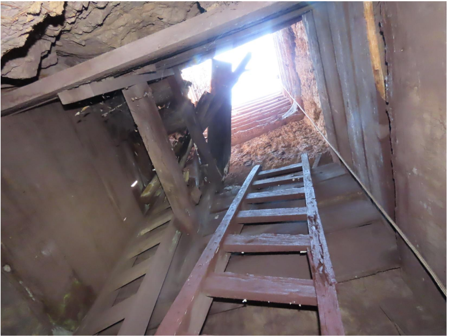
Homick Energy Maggie Mine Shaft: View from the shaft bottom looking up towards the surface. BCI Photo by Dillon Metcalfe
