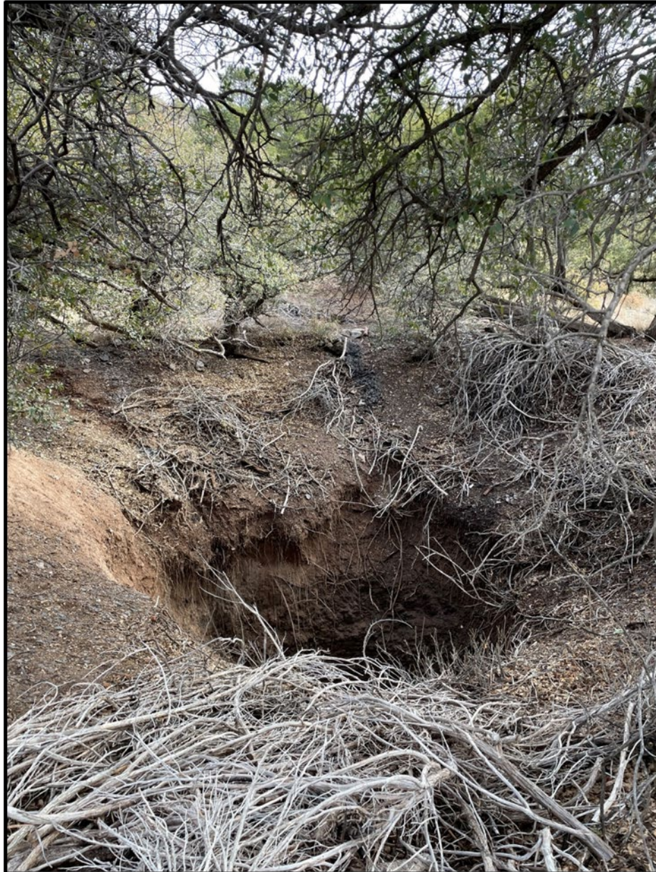
Figure 2.) Subsidence/Shaft – LA 54916 Feature 4: Facing South
