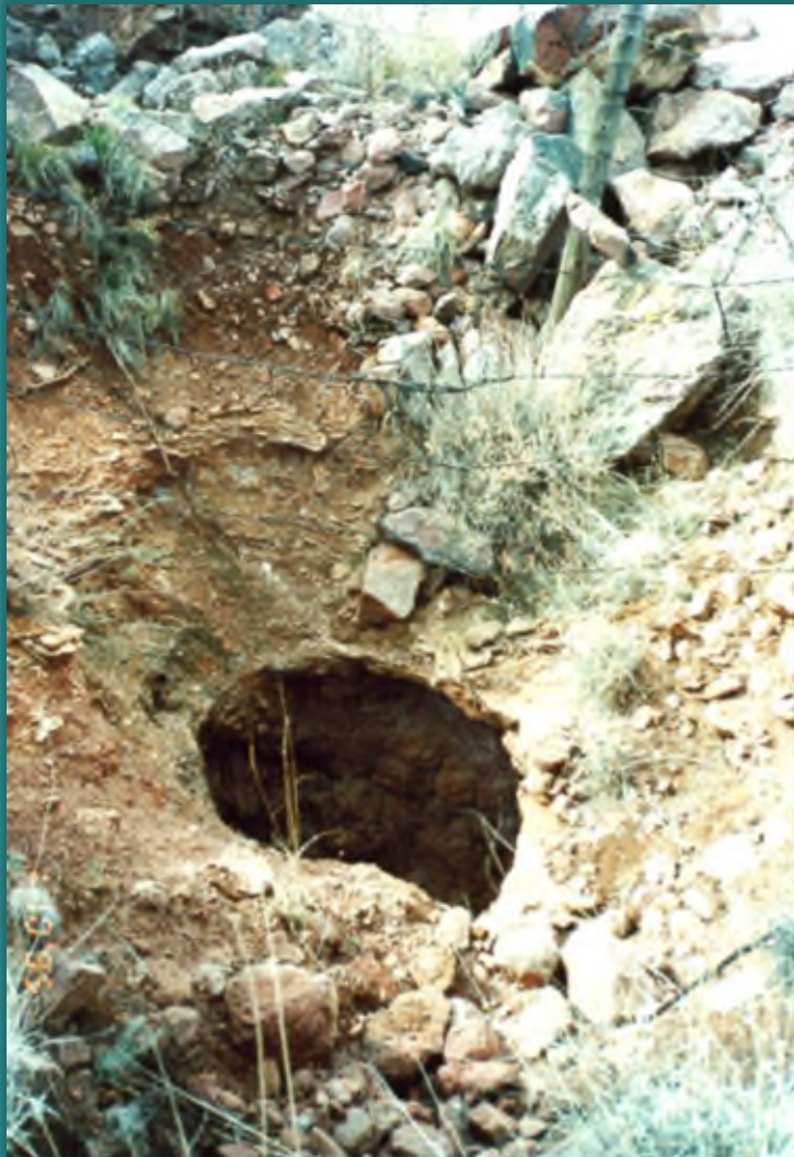
Before/After stope closure with rock-lined basin: Socorro West Mine Safeguarding – Photos Courtesy of AML
