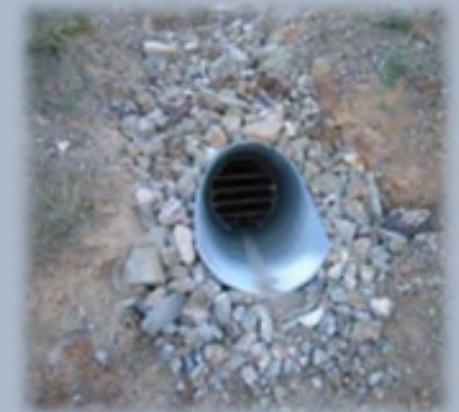
Culvert with Bat Gate
