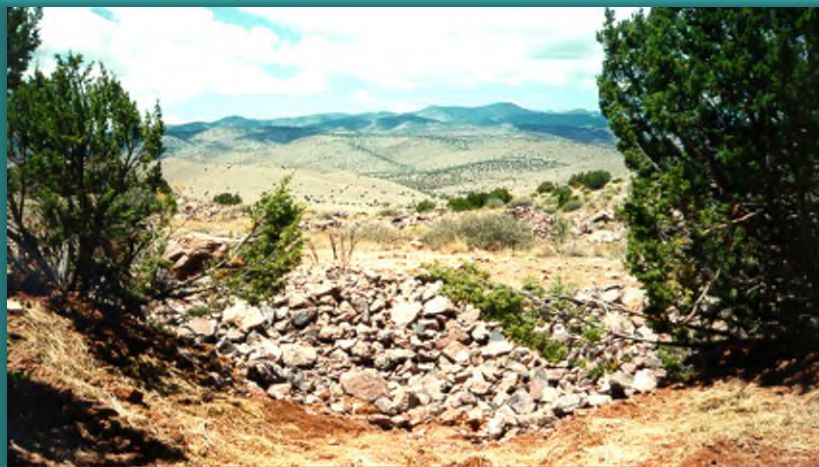
Before/After stope closure with rock-lined basin: Socorro West Mine Safeguarding – Photos Courtesy of AML
