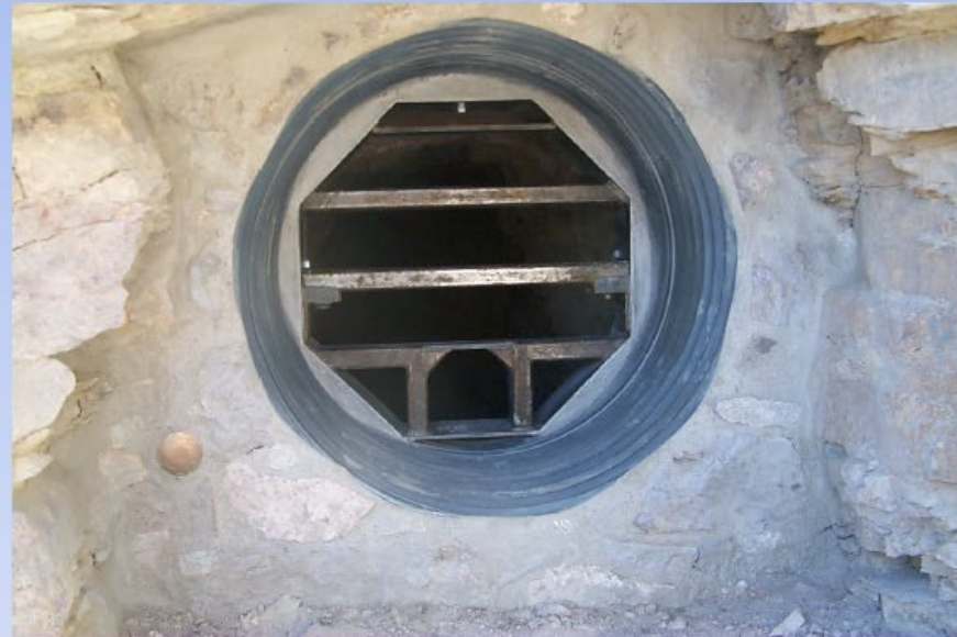
Culvert with bat and wildlife-friendly gate
