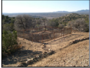
Steel fence enclosure around a partially filled shallow shaft
