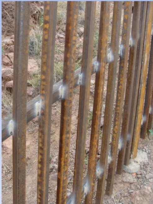
Closeup of typical weathered steel picket fence.
