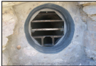
Culvert with bat and wildlife friendly gate
