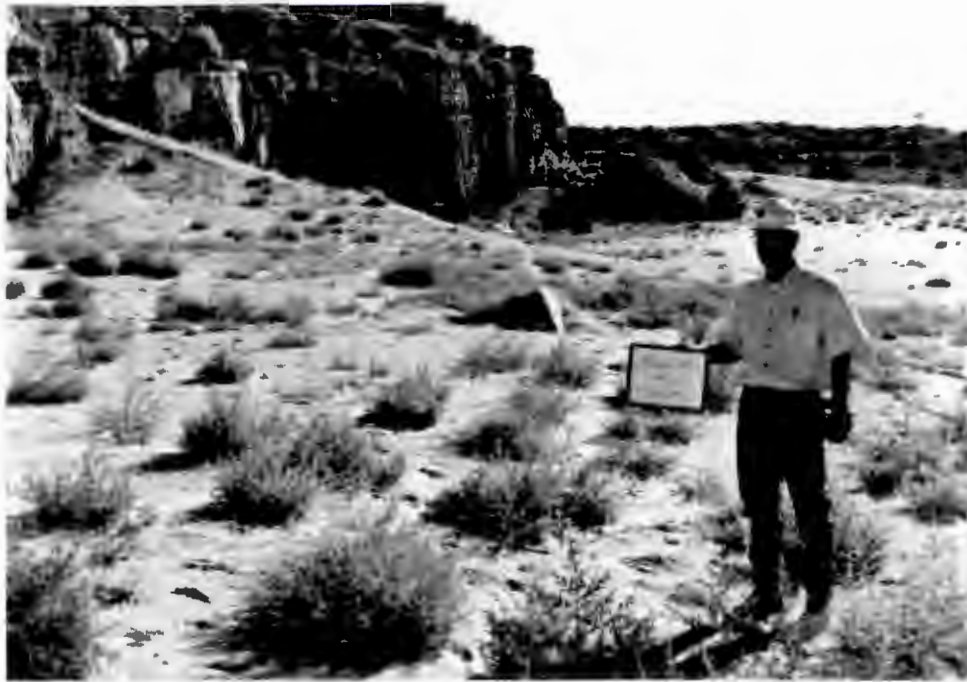
Marquez Mine, Reclaimed Declined Shaft, 9/12/95
