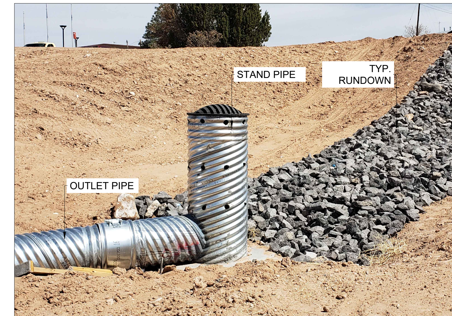
3 BETHLEHEM POND AND STANDPIPE INSTALLATION TYPICAL
