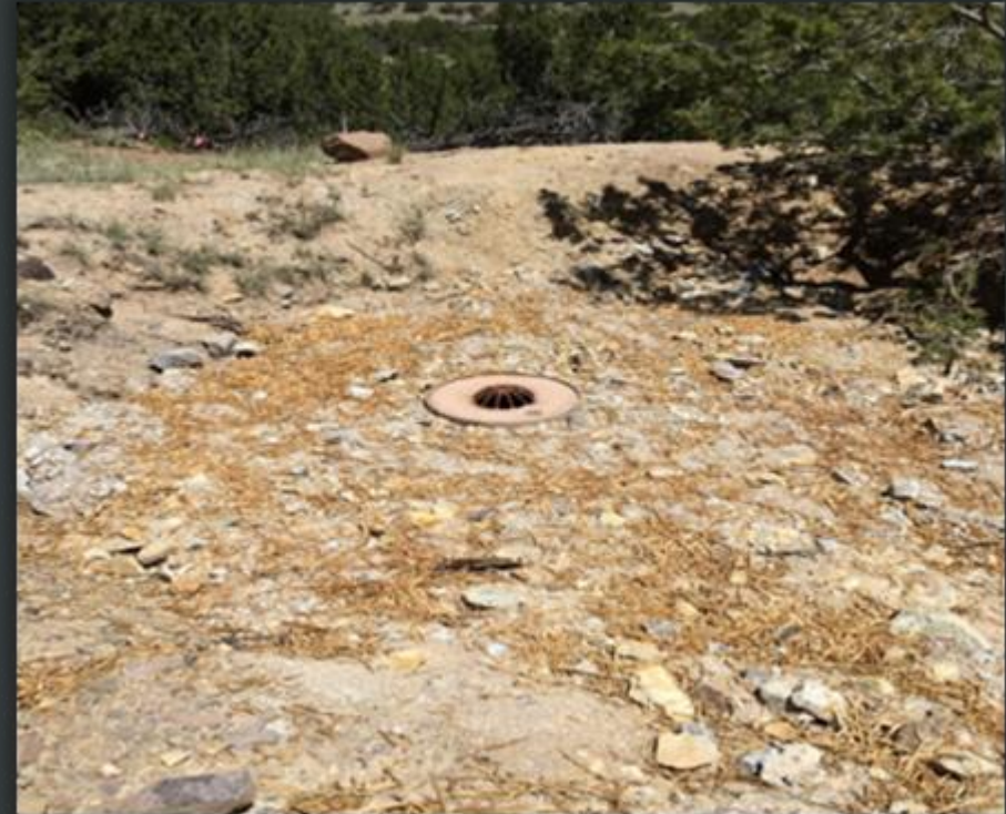
Polyurethane foam closure with drainage cap – Photo Courtesy of AML
