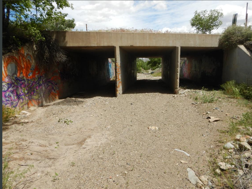
Channel with box culverts
