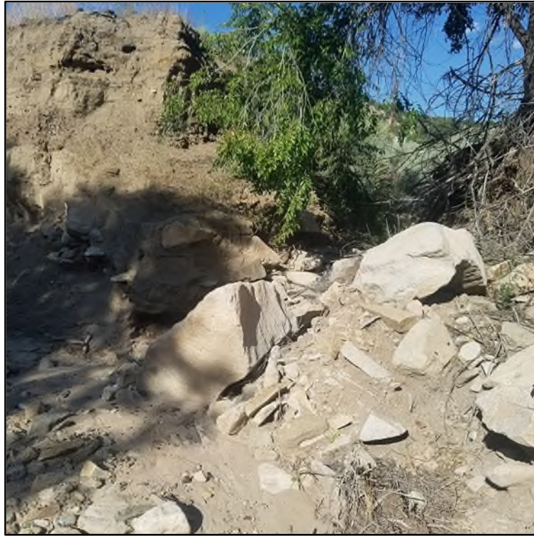
Figure C.3. DR02 convergence with DR01 facing upstream in the northern section of the APE (photo direction - southwest)
