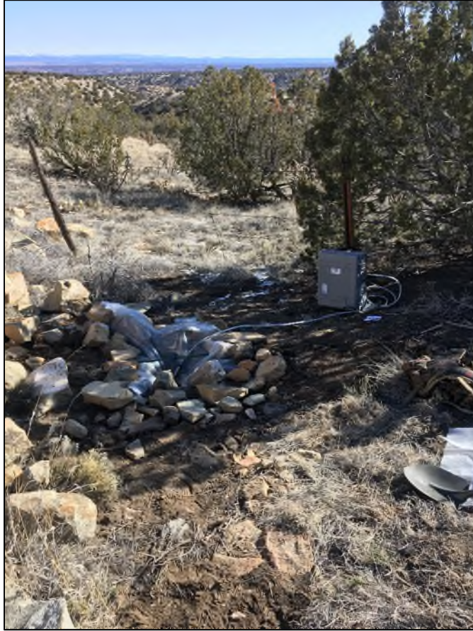
Water Quality Monitoring Site REF located on a hillside near the eastern edge of the Madrid APE
