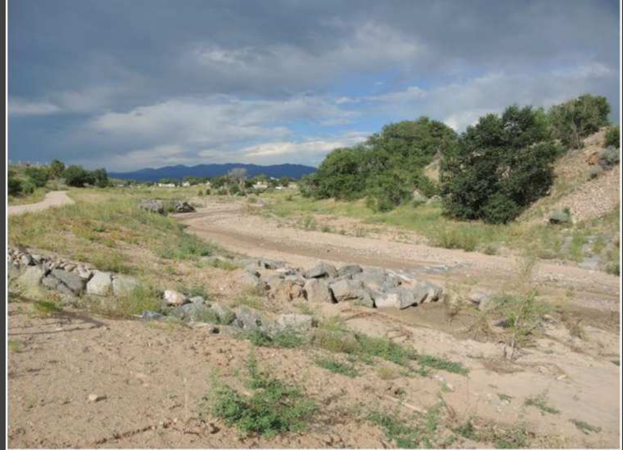
Arroyo and floodplain grading: meandering low-flow channel with adjacent floodplain, emergent willows at bankfull elevation.
