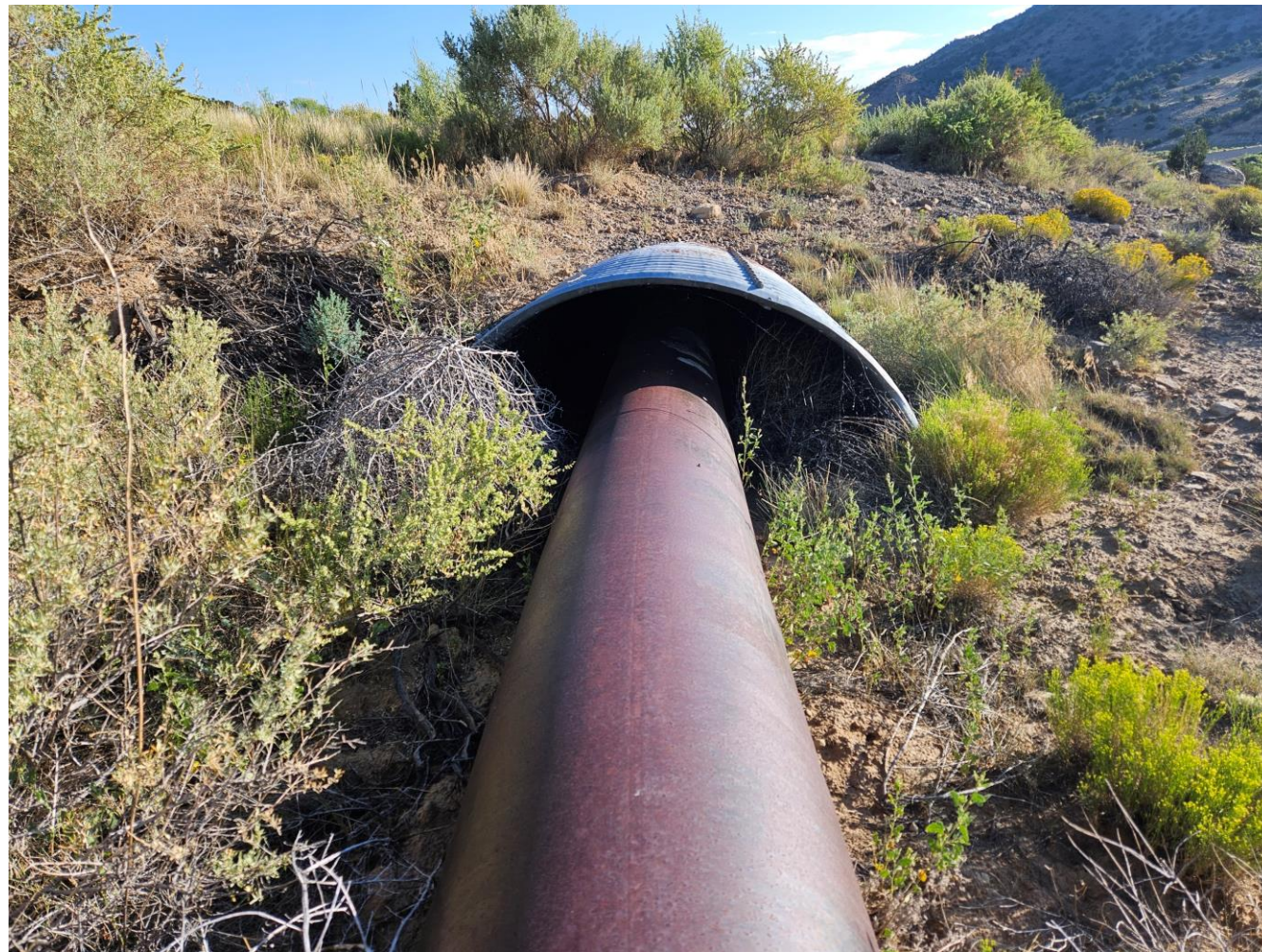
Pipe in CMP Crossing, County Rd 75 Crossing
