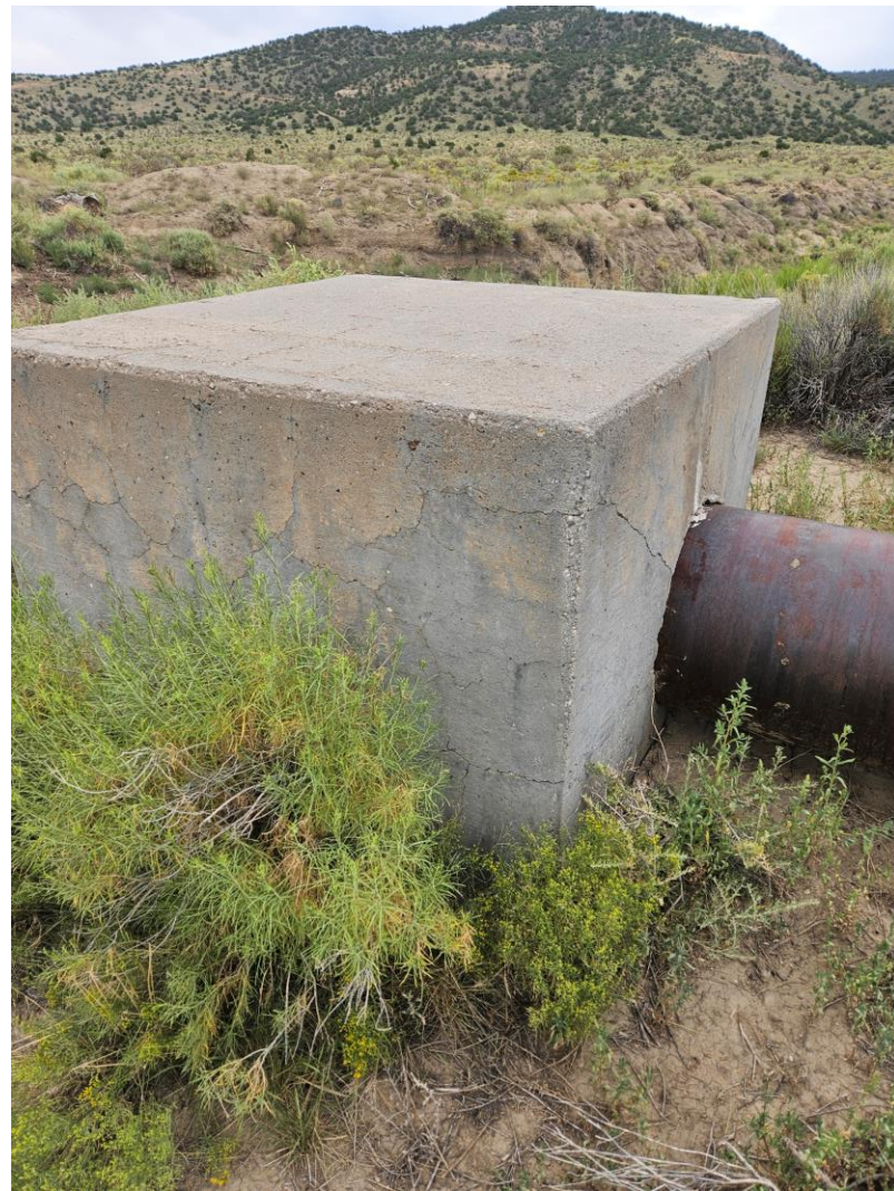
Thrust Block Example
