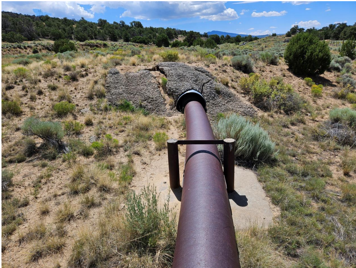
Pipe in CMP Crossing and Steel Anchor Structure in Concrete
