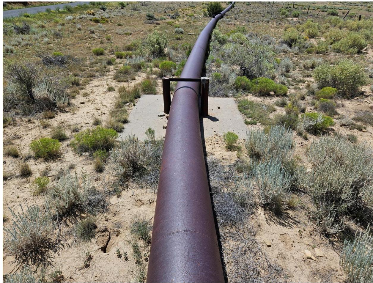
Steel Anchor Structure in Concrete with Metal Bollards
