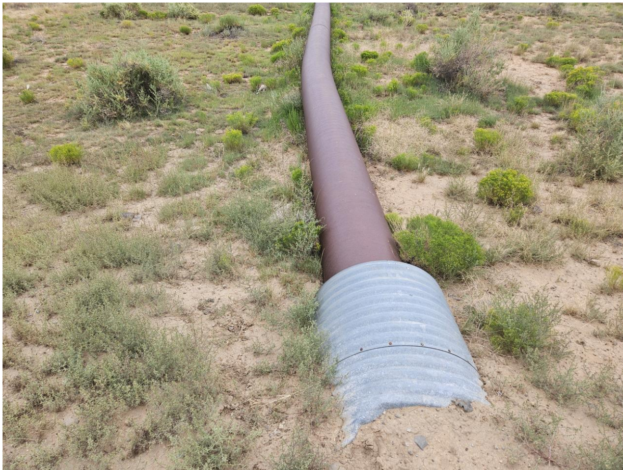
Pipe in CMP Crossing
