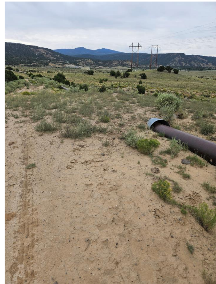
Pipe in CMP Crossing
