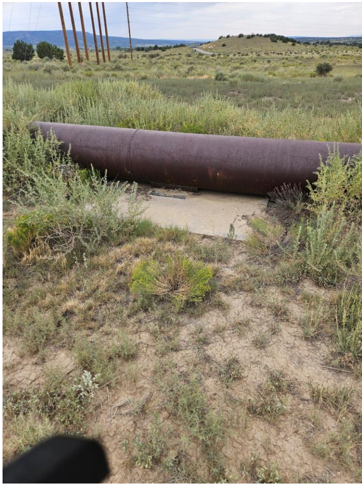
Steel Plate Welded into Pipe and Bolted in Concrete
