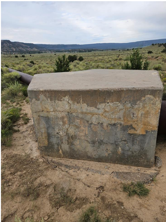
Thrust Block Example
