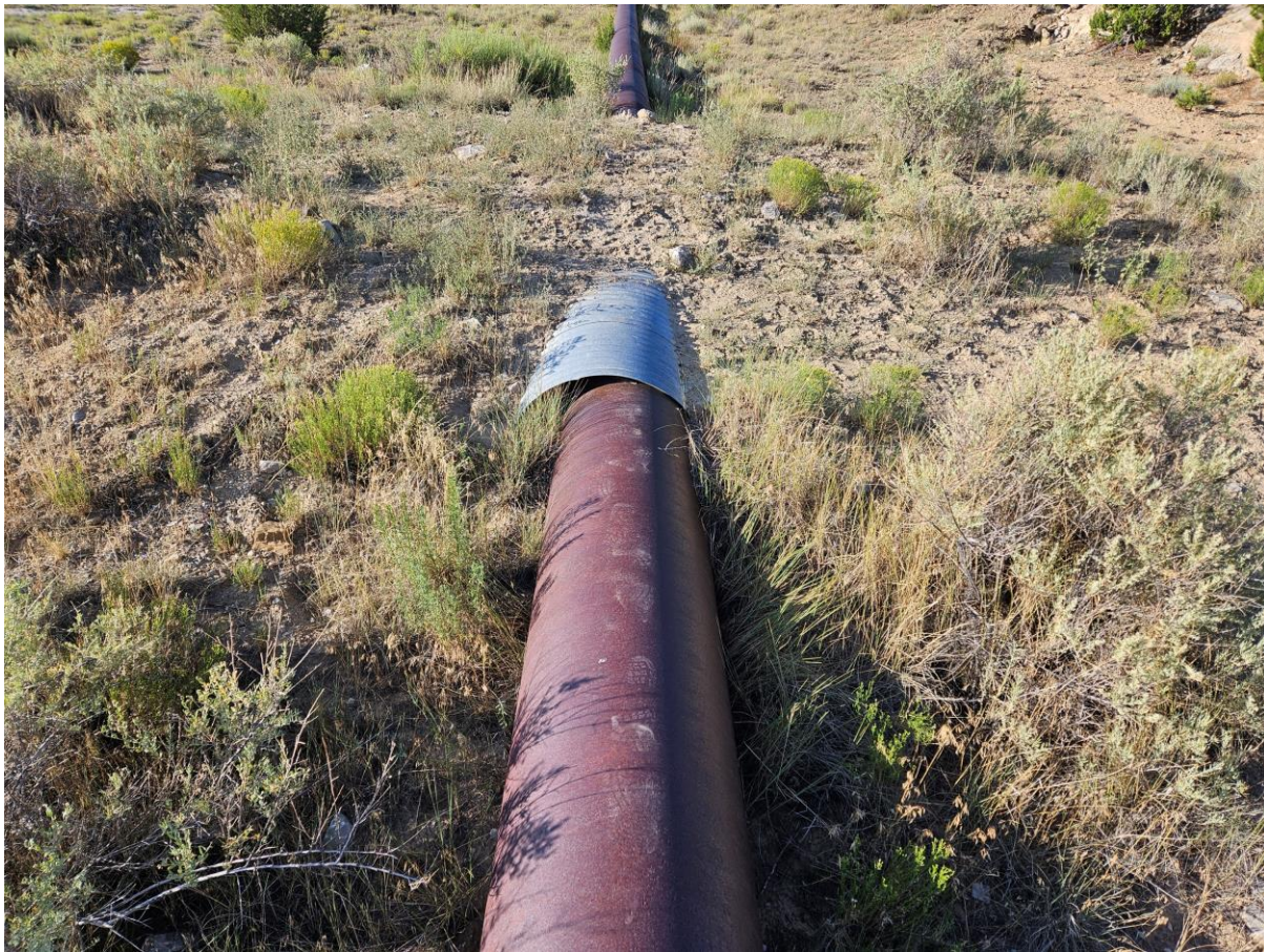
Pipe in CMP Crossing, Access Road Crossing
