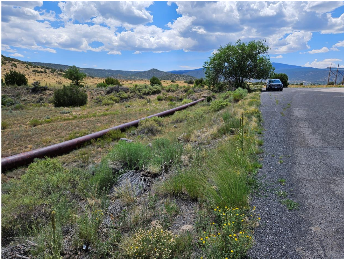
Pipe in CMP Crossing in USFS Hard-to-Access Area
