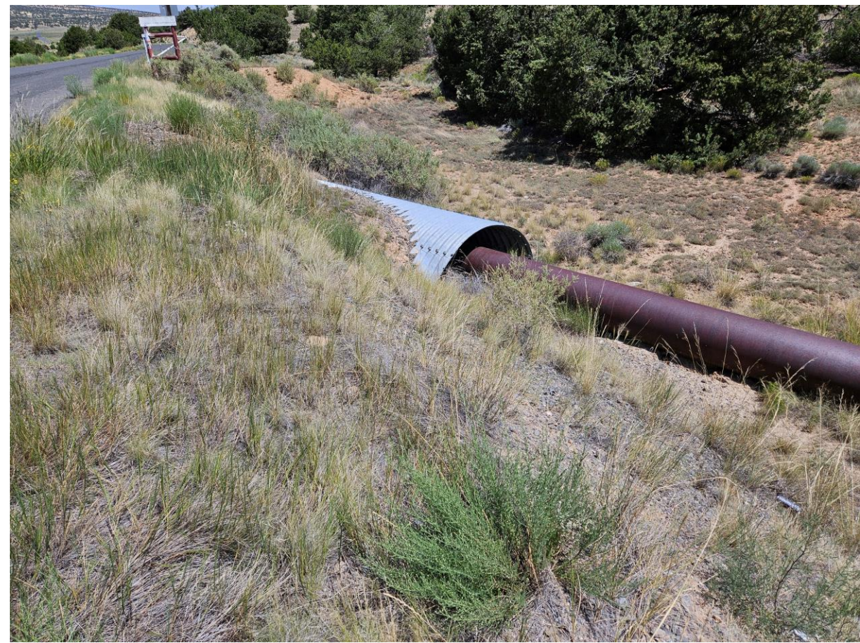
Pipe in CMP Crossing, Crossing County Rd 75
