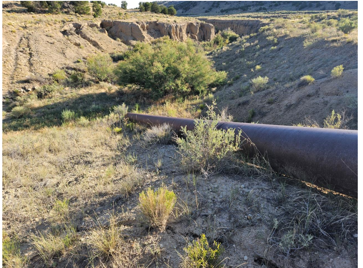
Last Segment of Pipe Buried and Point of Discharge
