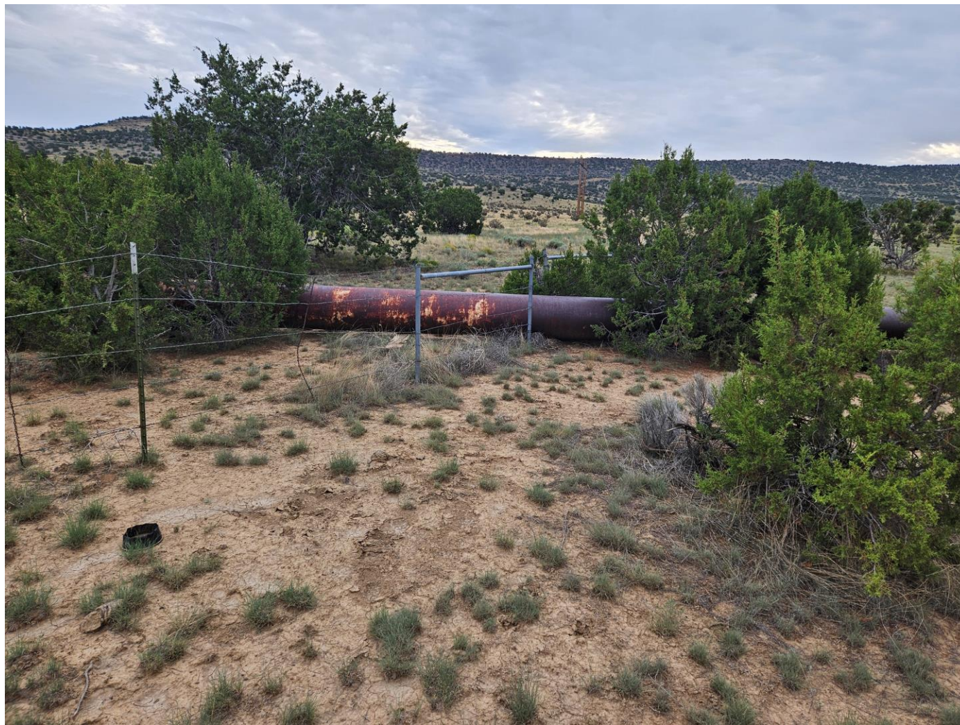
Pipe Crossing USFS Fence
