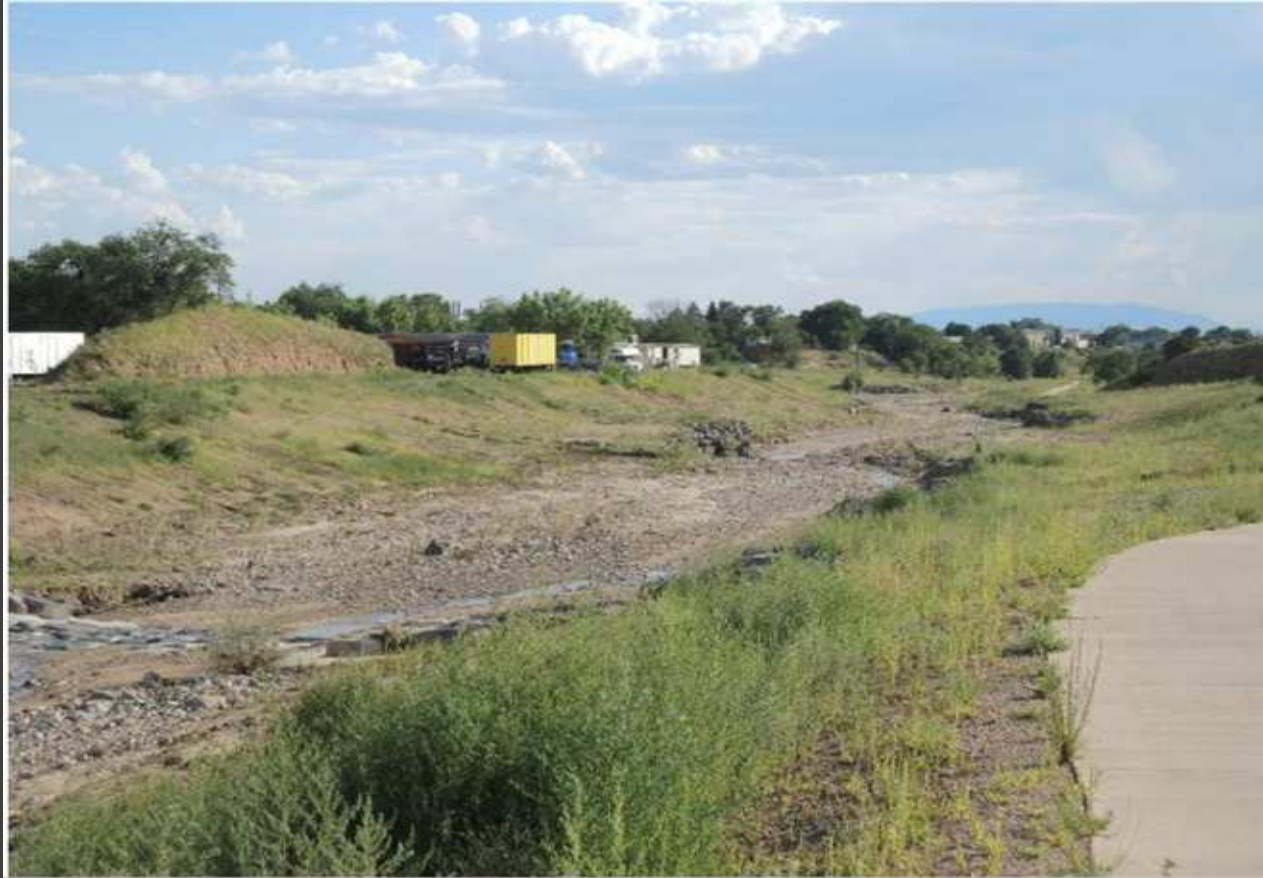
Arroyo and floodplain grading: meandering low-flow channel with adjacent floodplain, infrequent stacked boulder deflectors to manage channel migration and grouted boulder grade control structures to control channel bed elevations.
