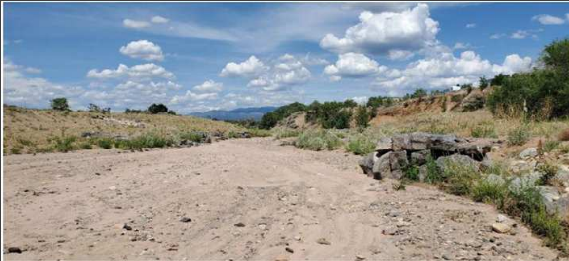
Arroyo morphology is laterally managed with rock structures and riparian vegetation.
