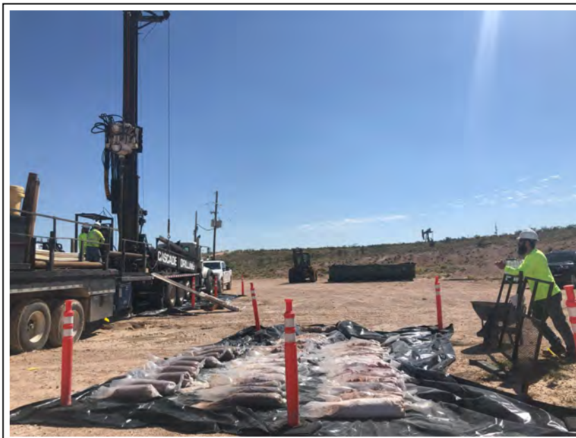
2. Sonic drilling at WDW-3-BH-1, October 5, 2023
