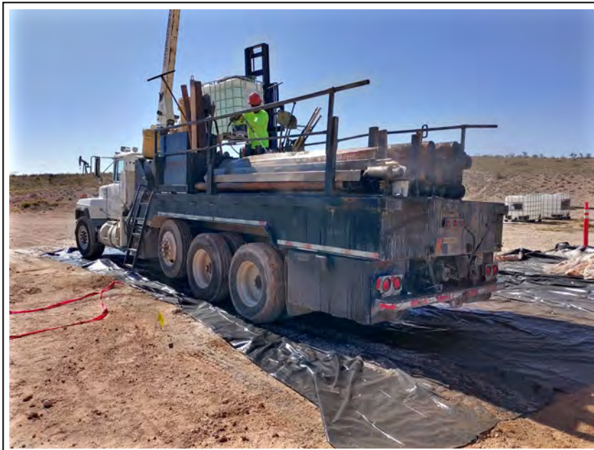
4. Rig decontamination
