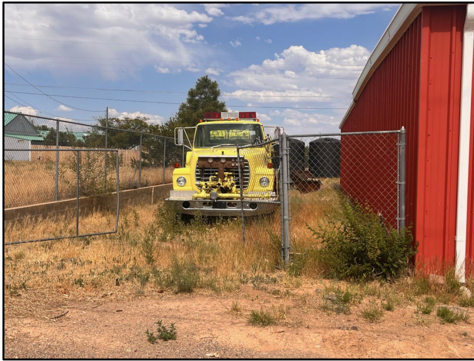
Figure 2.11. Example of a water catchment.
