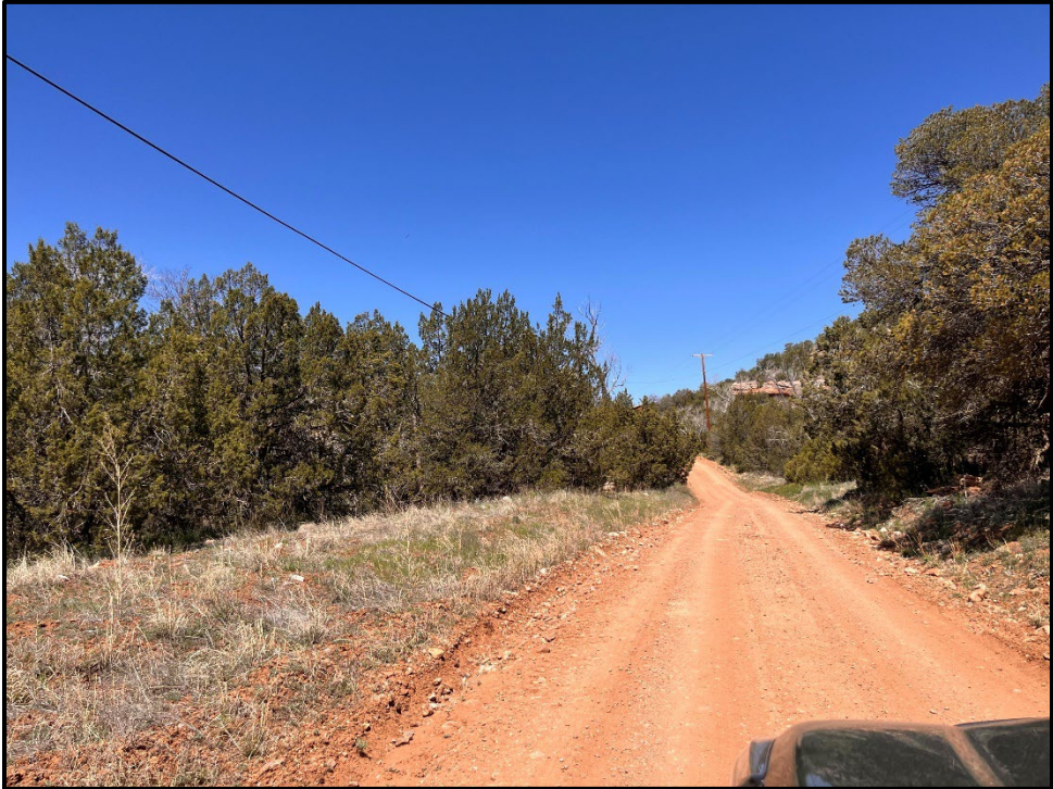
Figure 2.9. Example off on an unsurfaced road with dense vegetation on both sides.
