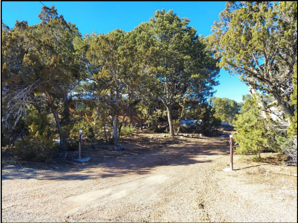
Figure 2.10. Example of an unsurfaced road with overhanging vegetation.
