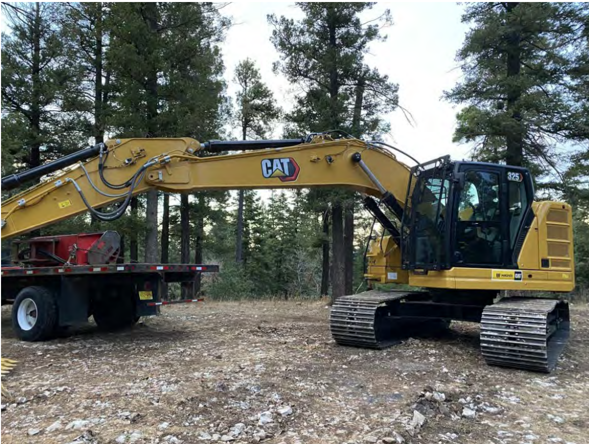
Equipment staged to begin work on the Sixteen Springs Project, November 2023.
