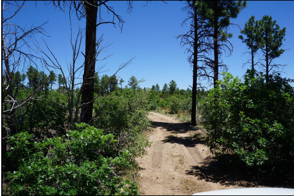
Figure 2.11. Example of a narrow unsurfaced road with limited turnaround ability.
