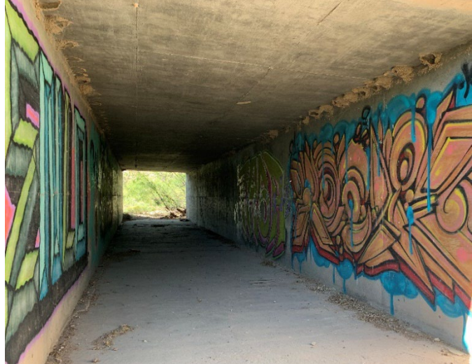
Figure 38: Box Culvert located on SLO property.
